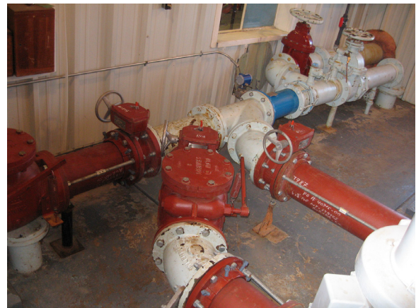
Figure 4. V-2 System Installed In A Tight Fit
